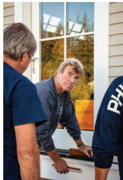
Steve Thomas confers with carpenters helping with his home renovation.
